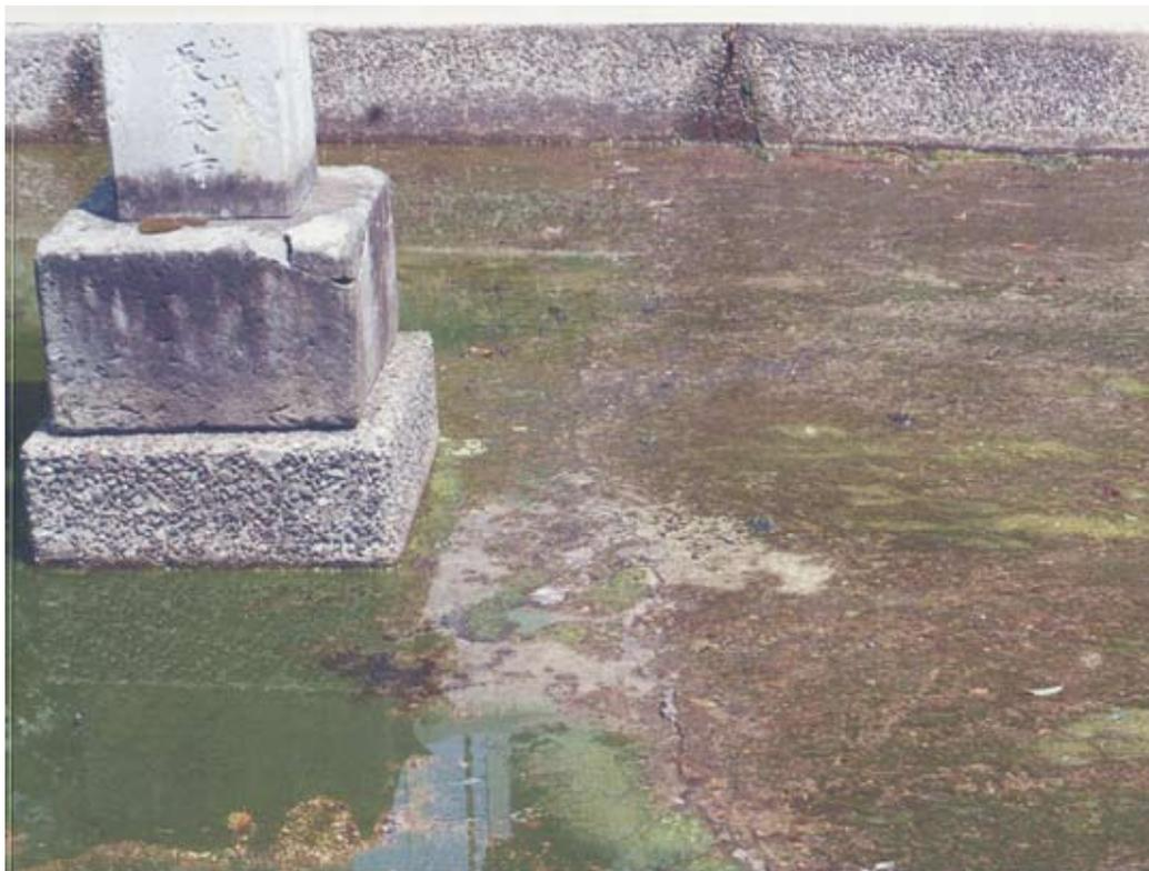
Fig.4 Crusher line of botom and side wall in pound.
